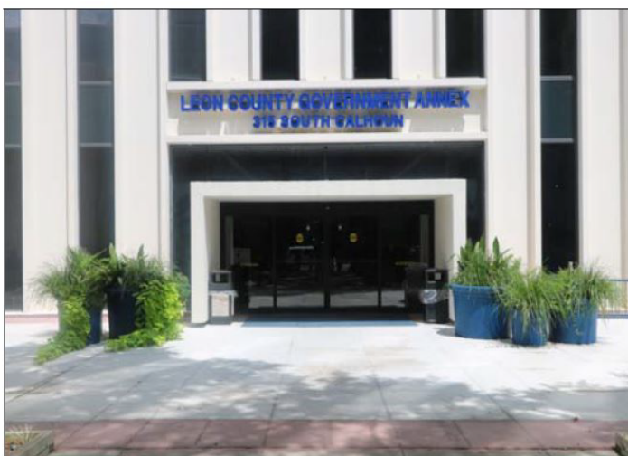
Leon County Government Annex Building
