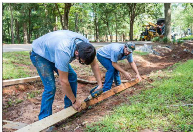
Construction of sidewalk for Community Safety & Mobility
