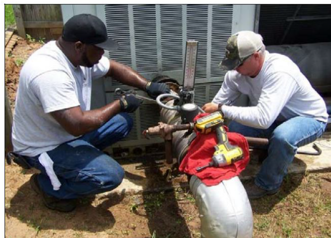
Building Mechanical Repairs and Improvements
