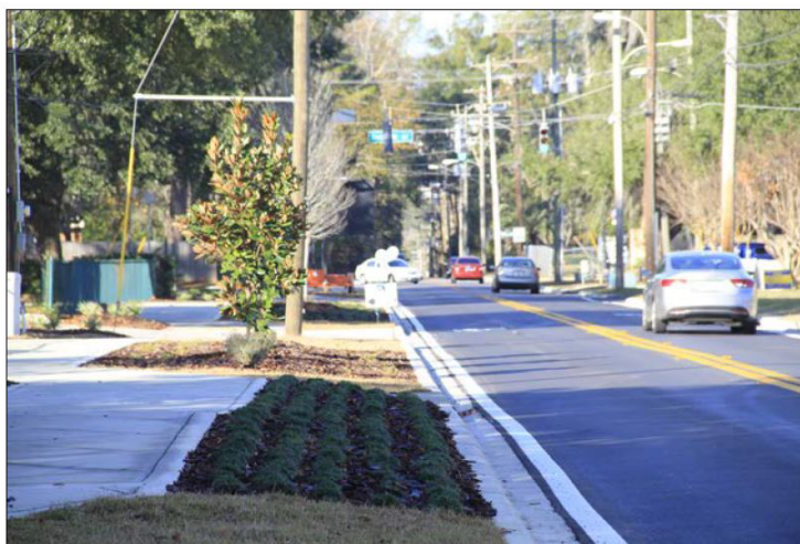
Roads Pavement Markings
