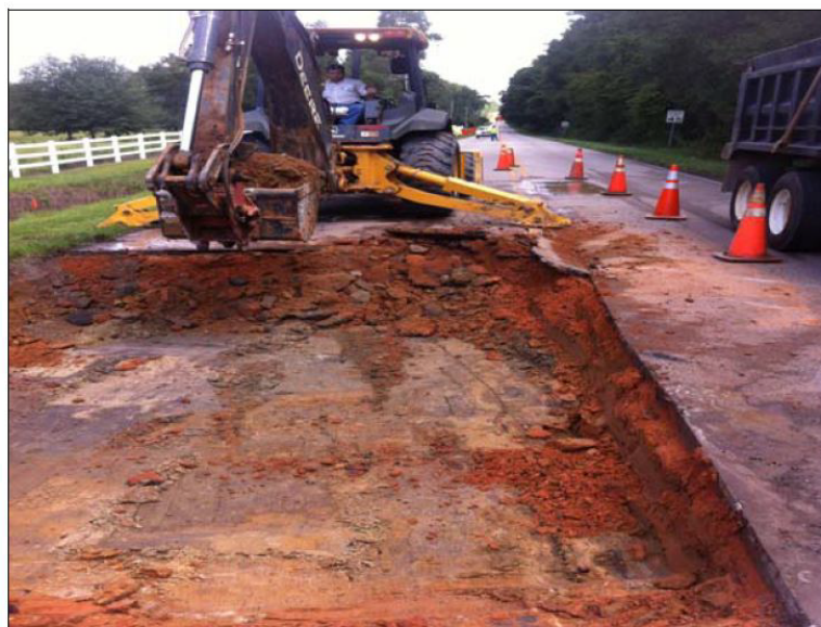
Asphalt Road Maintenance
