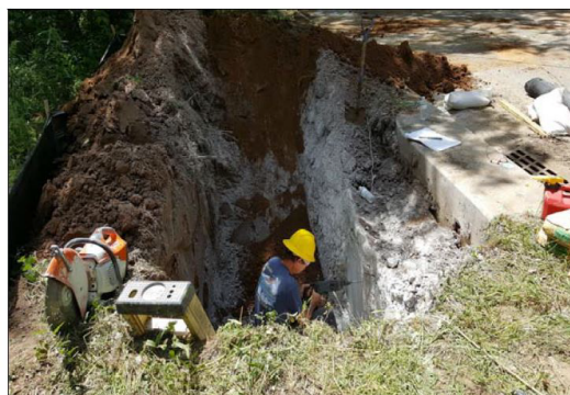
Stormwater Infrastructure Preventive Maintenance
