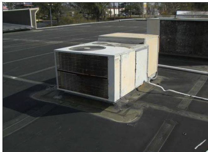
Building Roofing Repairs and Replacement
