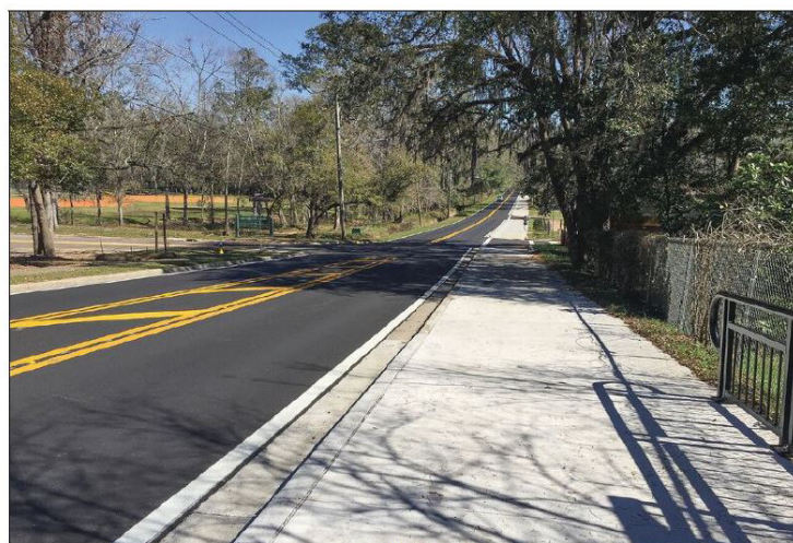
Local Road Resurfacing
